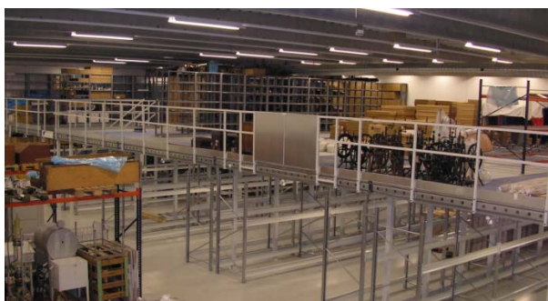
Figure 3 Picture of the interior of the museum storage showing the mezzanine construction (Photo Conservation Centre).
