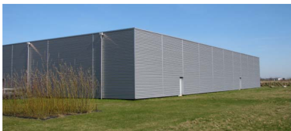
Figure 2 Exterior view on the main storage building after completion (Photo Christensen).
